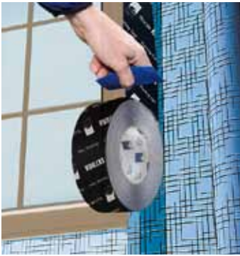
Apply TESCON EXTORSEAL sill tape to wall openings
