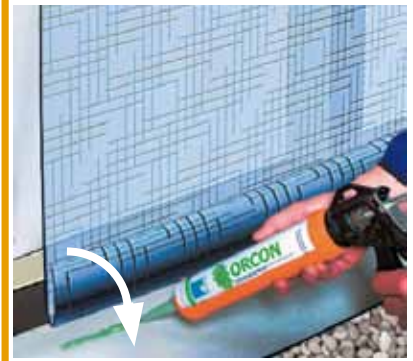
Use pro clima ORCON to adhere the SOLITEX EXTASANA to rough adjoining structural components or mineral surfaces.
