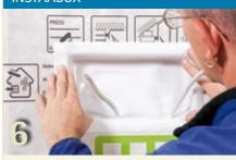
The airtightness box for power points and light switches is cut and fitted into the INTELLO® layer and then sealed by using TESCON VANA to create a seamless airtightness system.
