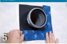
ROFLEX pipe grommets are affixed using TESCON VANA. Press firmly to secure the adhesive tape.
