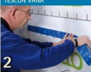
Seal the membranes at overlaps without strain or loading, using TESCON VANA adhesive tape. The tape should be applied centrally and pressed down firmly using, for example, pro clima PRESSFIX.
