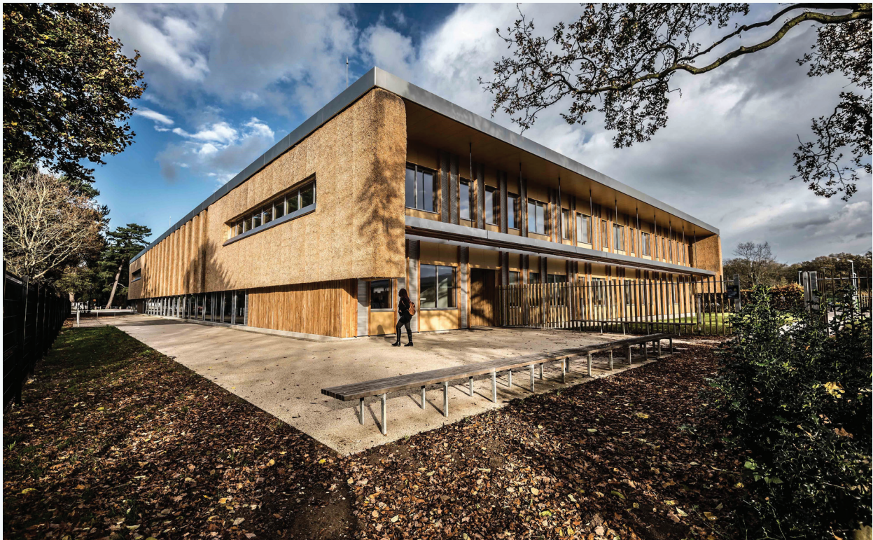
Figure 5. The Enterprise Centre, University of East Anglia, England, 2015, by Architype (UK) (Image: ©Photo by Darren Carter, Morgan Sindall)
